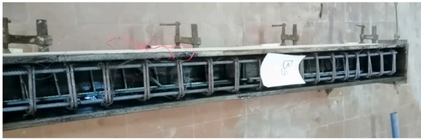
Fig. 3. Wooden form and reinforcement details of the test beams.
