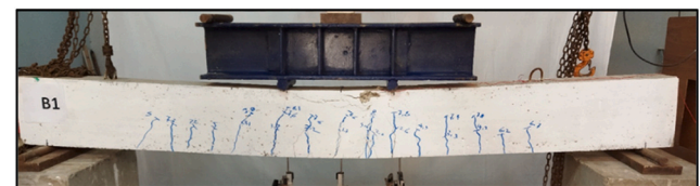
(a) Crack Patterns for the Tested Beam B1
